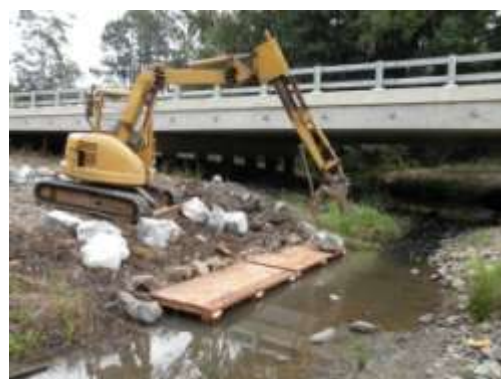
LUNKER installation, Belli Creek
