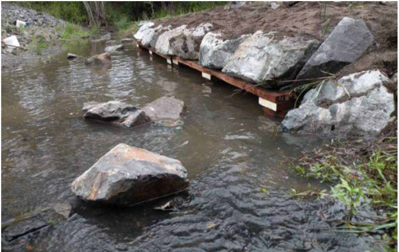
Installed LUNKERs at Belli Crossing 2
